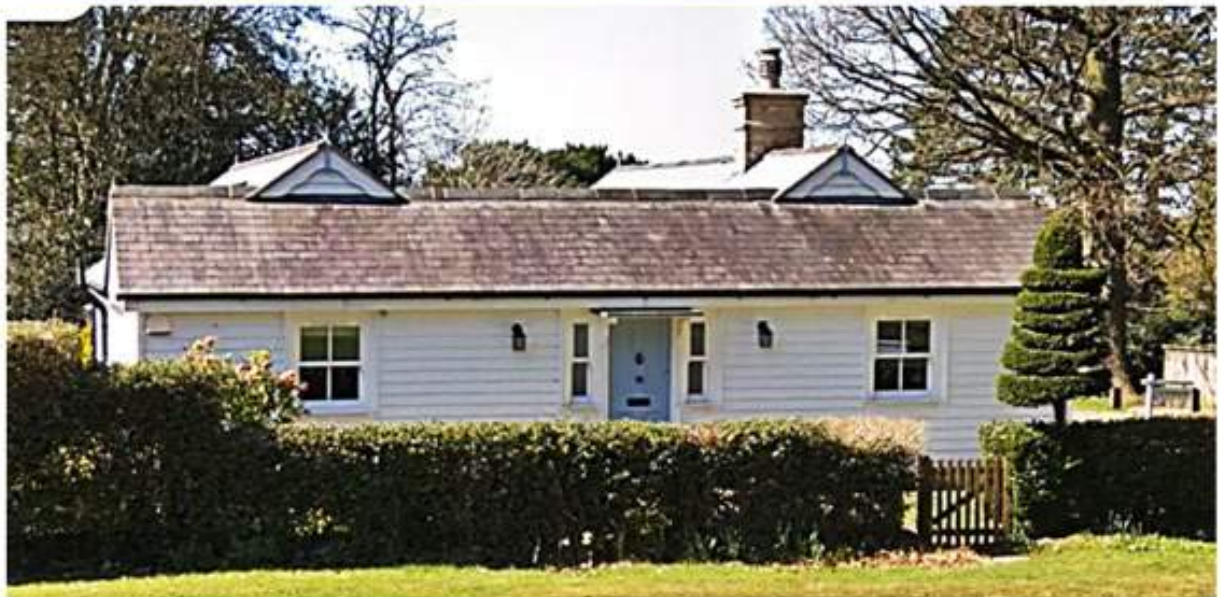
The Bungalow Locally Listed Building late 19 th century cottage constructed from railway shed
