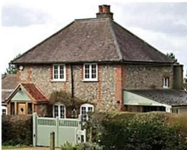
Holly Cottage 17 th century Locally Listed Building
