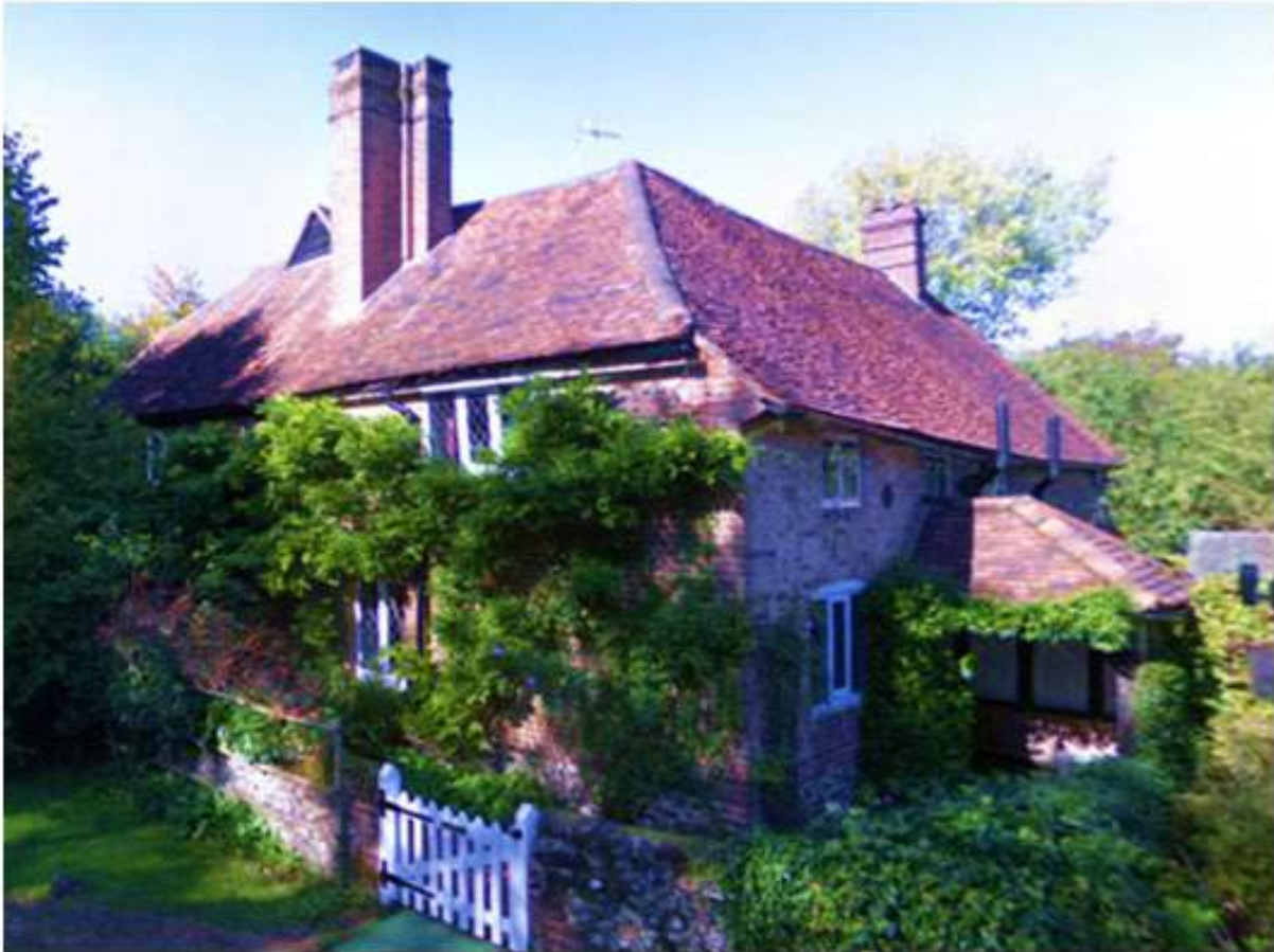
Hazelwood Farm 15 th century grade II listed Building Source Google Streetview
